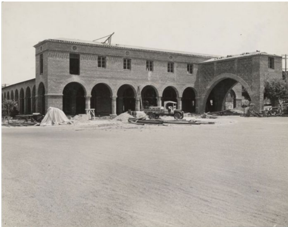
Figure 4 Syndicate Building under construction, 1929 (Palos Verdes Homes Association)
